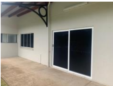
New security door
